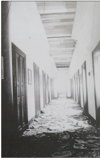
FIGURE 3. Damage in the Governorate Palace, the main Vatican administrative building, after the November 1943 bombing of the Vatican. Photo by Luigi Felici, Vatican photographer. Repr. in Augusto Ferrara, 1943: Bombe sul Vaticano (Vatican City, 2010). Photo reproduced by permission of the author.
